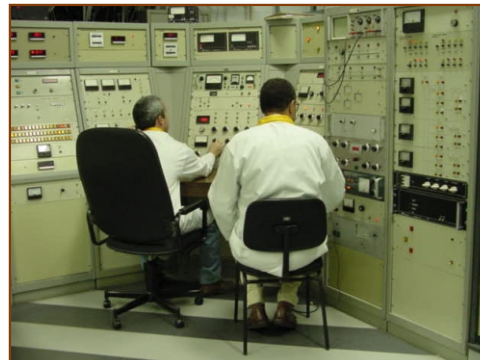
FIGURE 1 - Control room of the cyclotron CV-28.
