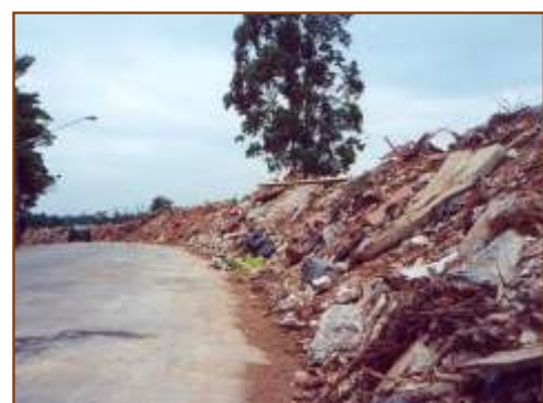
FIGURE 3 - Irregular disposal in S.Paulo south region.
