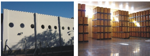
Figure 5. New radioactive waste storage building (outside and inside view)
